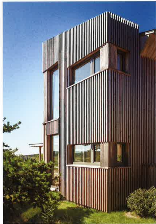
The exterior is clad in eastern hemlock (above). "It's local, it's native, and it's actually got a good bit of resistance," Winkelman says of the material, "and we could mill it to a unique dimension." The living room is furnished with a Tolomeo Mega floor lamp by Artemide, a Milo Baughman
