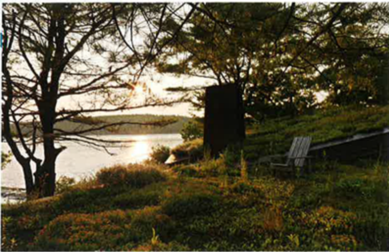
Planted mostly with sedum and grasses that are prevalent around the house, the roof requires little maintenance other than the occasional weeding and planting of supplemental material. A hefty copper chimney anchors the entry and reflects warm tones and light as it vents the woodstove.
