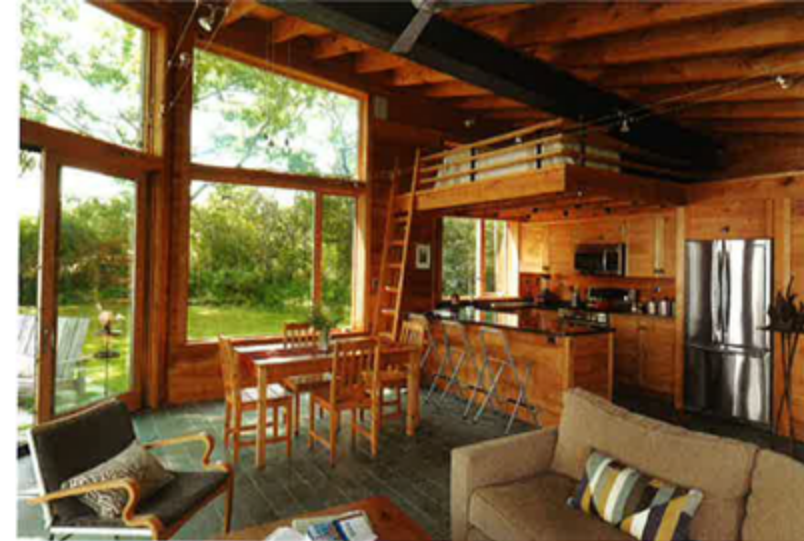
The open kitchen/dining/living space is awash with daylight and mostly locally sourced materials. The exposed rafters are hemlock; the wall finish is eastern white pine; and the floor is slate, chosen for both its capacity to absorb passive solar gain and to transmit radiant heat.
