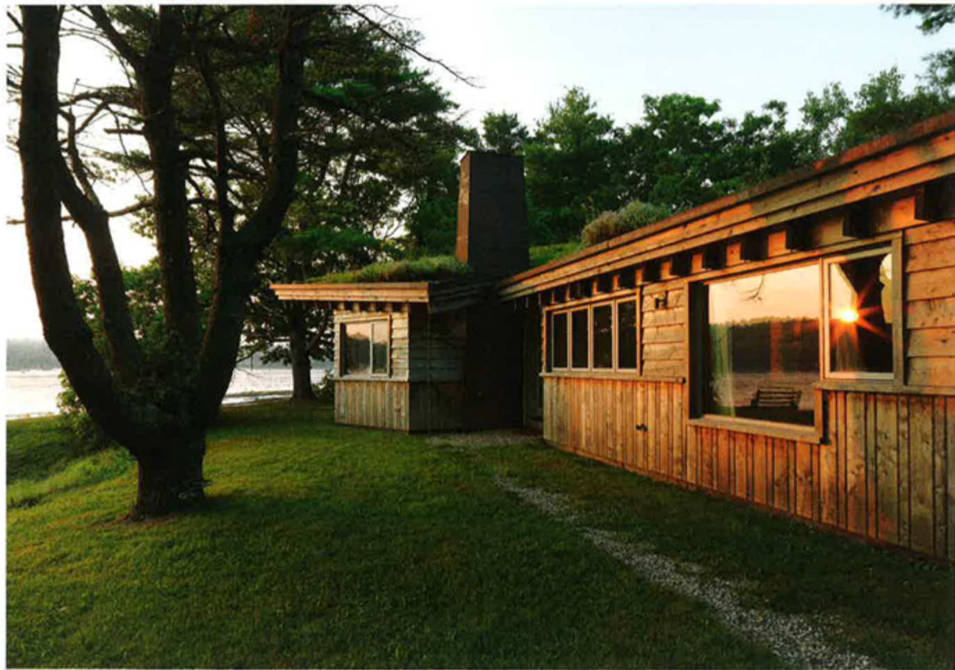
The 1-in. tamarack, a locally sourced material that's rot resistant and more affordable in long lengths than cedar, is arranged vertically, like wainscot, to suggest a base and then horizontally to emphasize the massing of the house and low-slope of the rafters. The 8-in. coursing relates to the wide trim dimensions on the eaves and is meant to reflect the rugged wood dimensions you find in nature.
